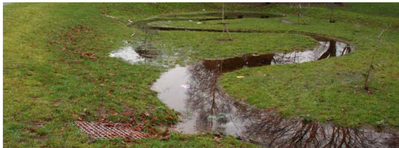
Controlled flows are released from one sub-catchment feature to the next, as here at Birchen Coppice Primary School, Kidderminster.
