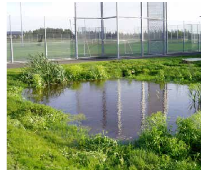
Pershore High School, Worcestershire. Swale conveyance into pond site control for final treatment and storage.
