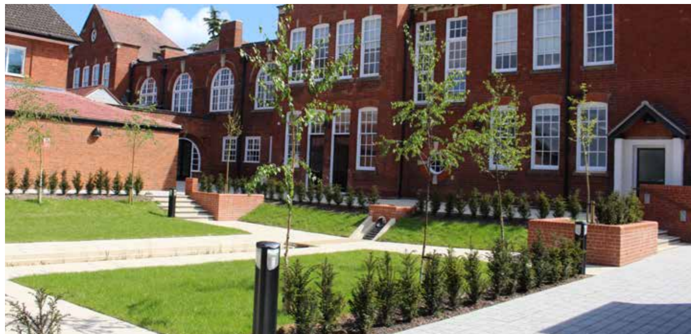
A sunken SuDS courtyard with solar water feature into a formal rill at Bromsgrove Civic Centre.
