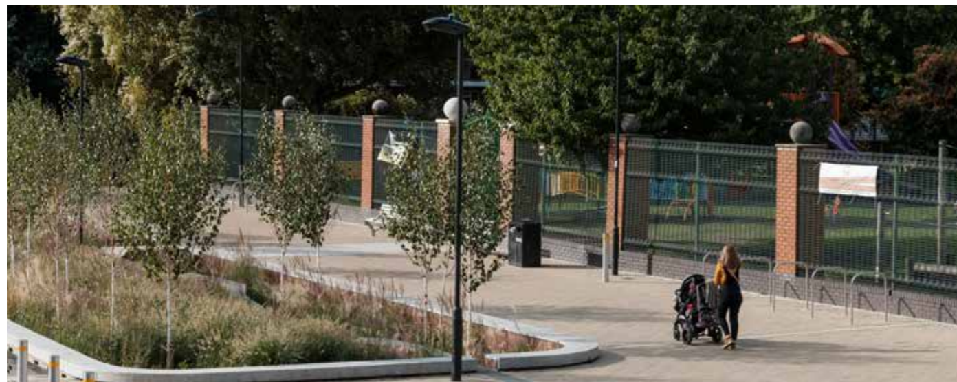
Australia Road, London, where permeable paving provides source control prior to SuDS Basins.
