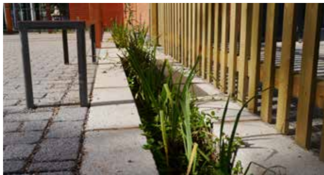
A planted rill at Bewdley School Science Block.
